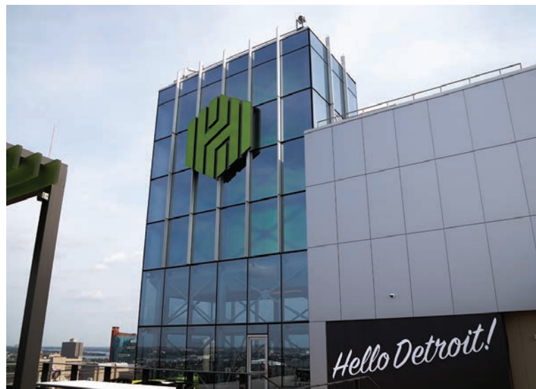
The new Huntington Bank headquarters in downtown Detroit is made up of 10 floors of parking space, 10 floors of office space and a rooftop deck. | QUINN BANKS/CRAIN'S DETROIT BUSINESS
